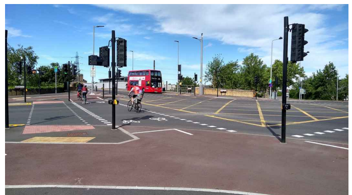
This junction has cycle crossings which adds signal heads. However, with a simplified layout and careful placement, the minimum of signals required for safe operation are provided.
