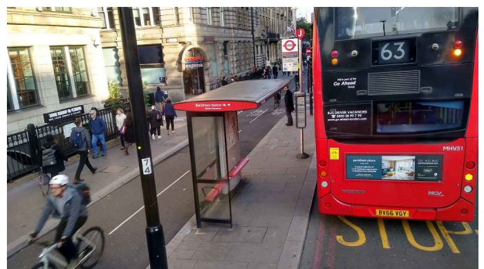
The floating passenger area here is not particularly wide and shelter proximity to the cycle track both creates a risk to people cycling clipping it and obscures the views between passenger and people cycling.
