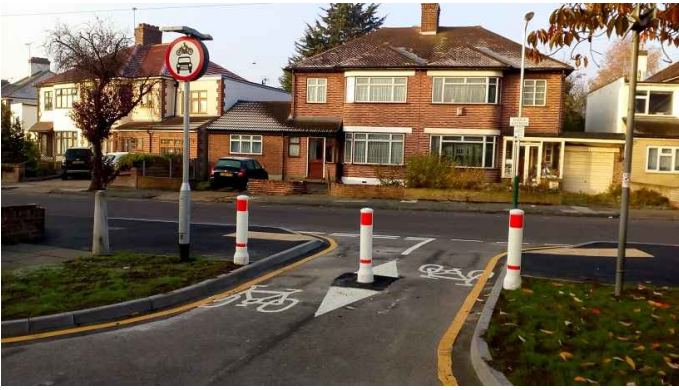
Access control using conspicuous overrunnable bollards with 1.5 metre air gap.
