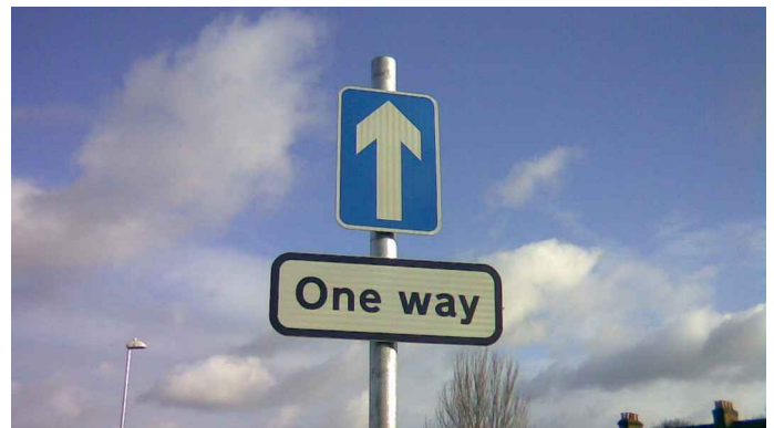
A one-way sign with a non-prescribed use of a plate below. Poor knowledge of signing rules is often a reason for sign clutter.
