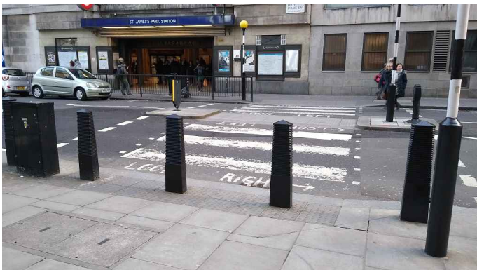
Bollards protecting a building (behind the photographer) interfering with a zebra crossing.
