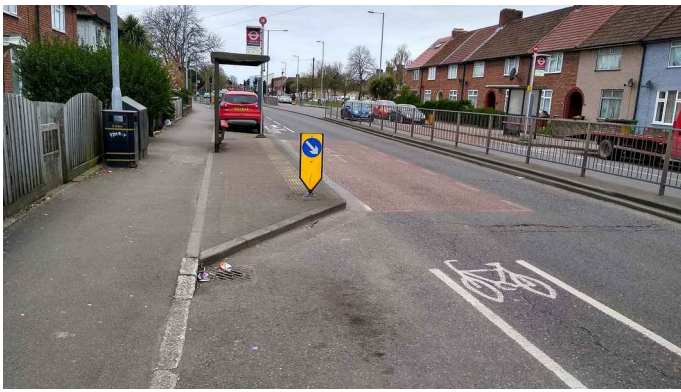
This build-out places the bus stop out from a line of parked vehicles, but it also provides space for a shelter and flag.
