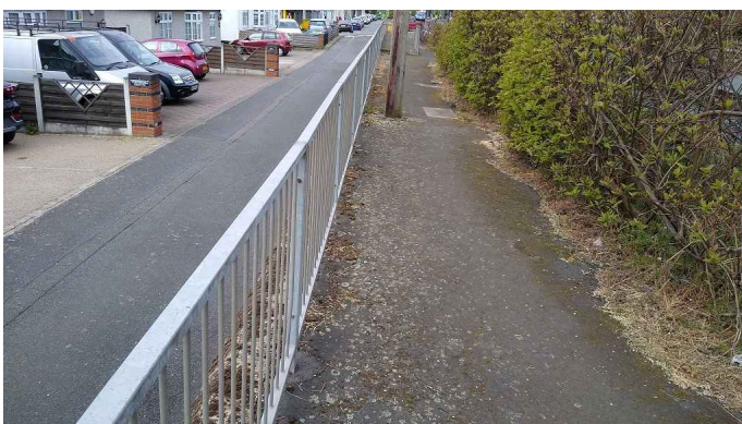
Guardrail being used where the carriageway is at a much lower level than the footway.
