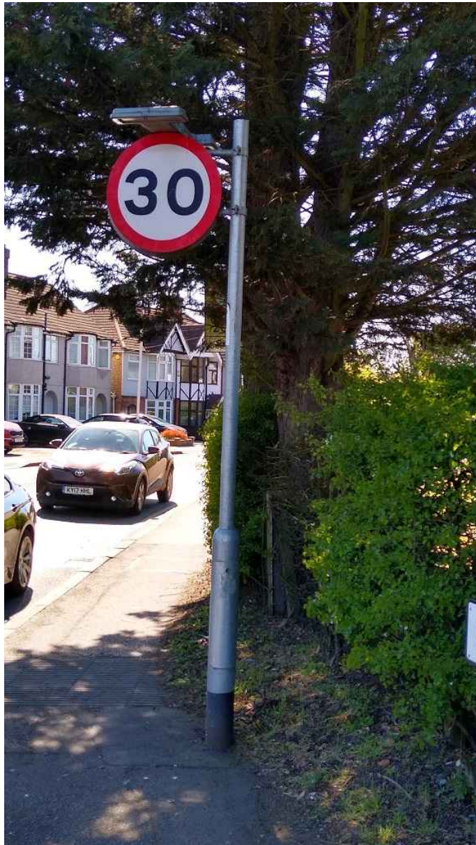
30mph “terminal” sign with the post at the rear of the footway to maximise footway width using a bracket system to “hang” it further towards drivers’ field of view.
