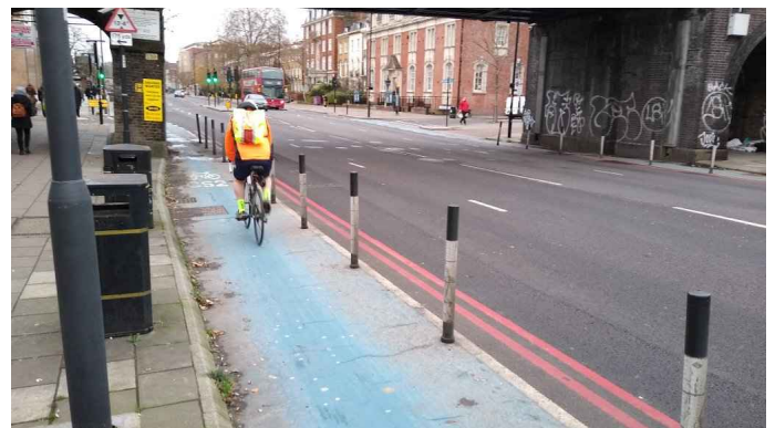
A wand-protected cycle lane Bow Road, East London. The wands present a continuous “wall” which reduces the effective width by 500mm and the bridge support provides another 500mm loss making it very narrow for cycle traffic to pass.
