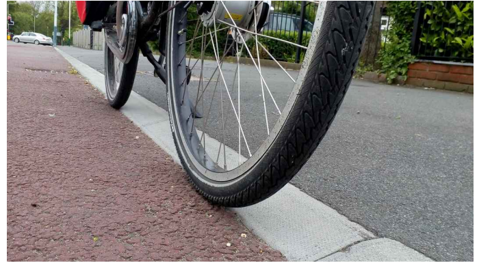
A gently sloping “forgiving” kerb between a cycle track and a footway allowing the full width of the cycle track to be used.
