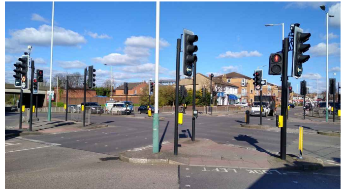
A junction with slip roads and multi-stage pedestrian crossings significantly increasing the number of signals.
