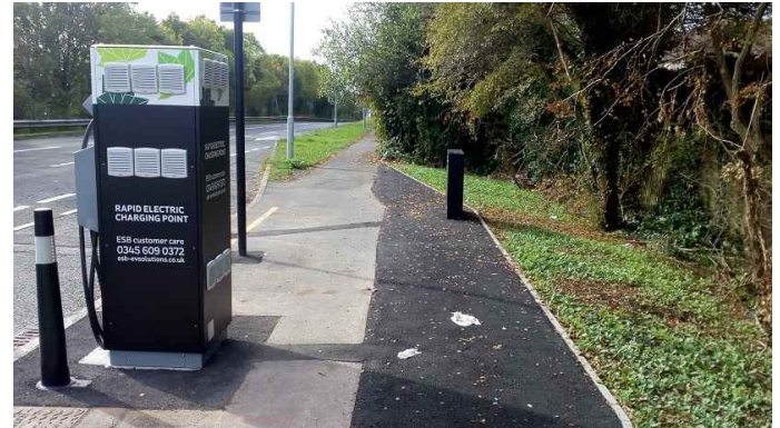
Rapid charger with a feeder pillar in the distance (on the right). The footway has been widened to compensate for the loss of space created by the charging unit.
