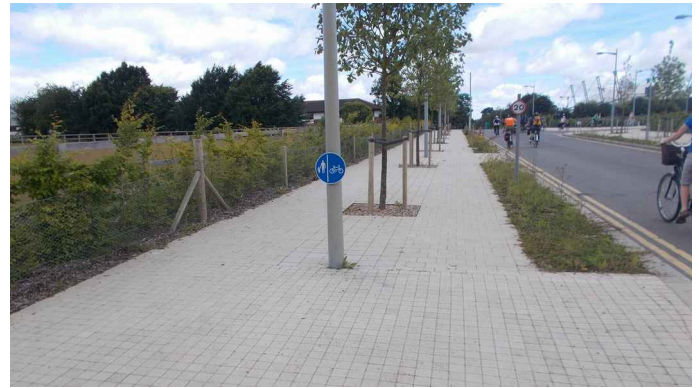
Ada Lovelace Road, Cambridge. A clutter line is used to demarcate walking and cycling space, although the materials don't provide delineation and users rely in signs. Having the trees and lighting columns in the verge would have given more walking and cycling space.
