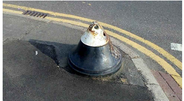
A bell bollard used on the corner of a tightly laid out junction.
