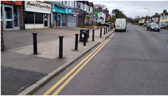
Bollards used to stop drivers parking on shop forecourts.
