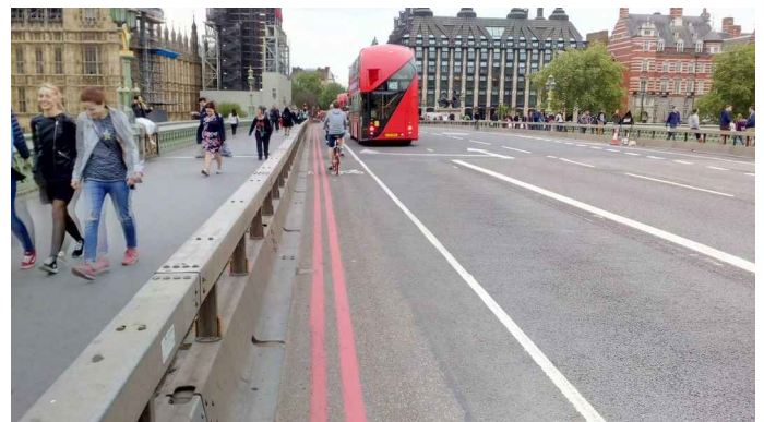
This steel barrier was placed on Westminster Bridge in London in the aftermath of an attack by someone driving along the footway and hitting people walking.
