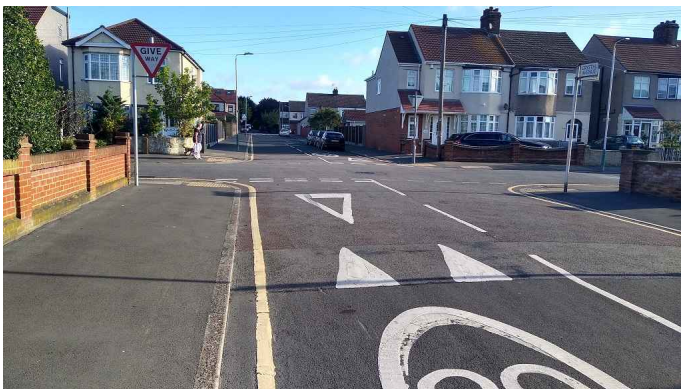
Give way markings, a triangle and an upright sign all being used within a traffic-calmed 20mph residential street. Inappropriate clutter.
