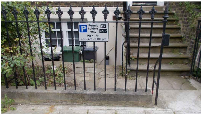
Parking bay sign attached to railings.
