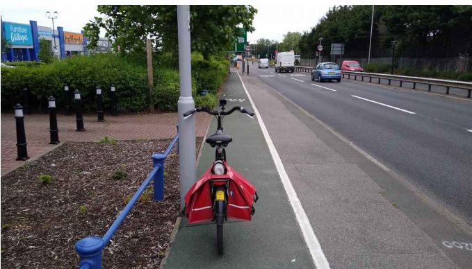
A lighting column placed at the edge of a cycle track creates a risk of “handlebar strike” which could easily cause the rider to fall. This should be 0.5m outside the edge of the cycle track.
