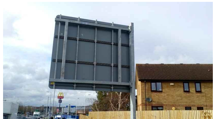
On the reverse side, the sign face is attached to a steel framework.
